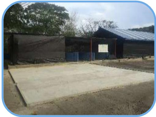
Figure 1: Concrete base for nursery including water outlet on the left.
